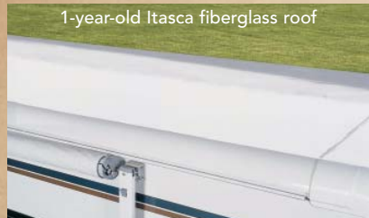
1-year-old Itasca fiberglass roof
